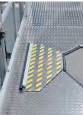
Service door in platform floor; anti-slip coating on underside
