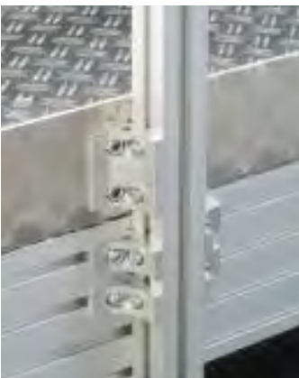
Post mounted to platform and angle used to attach baseboard
