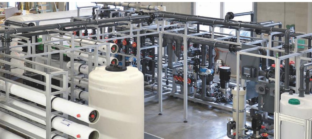
Flexible light-duty frame made from Series 40 profiles for desalination plant
