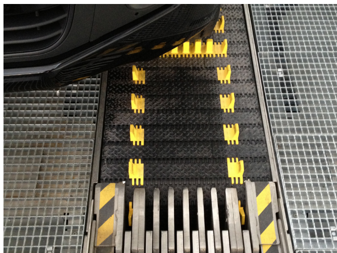
Exterior carwash entry 3125 belt conveyor with t2 pushers
