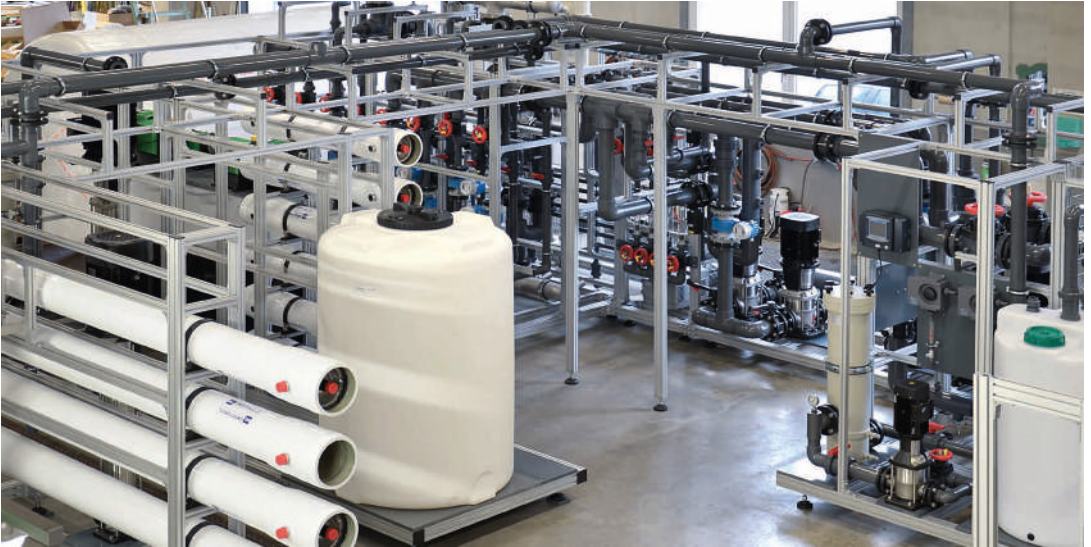
Flexible light-duty frame made from Series 40 profiles for desalination plant
